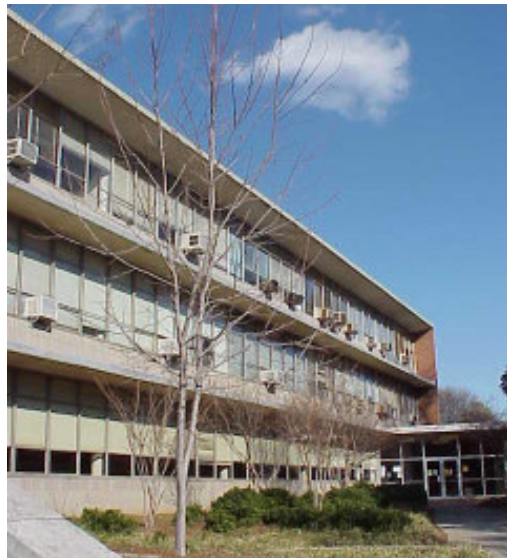
Hightower Building - south facade
